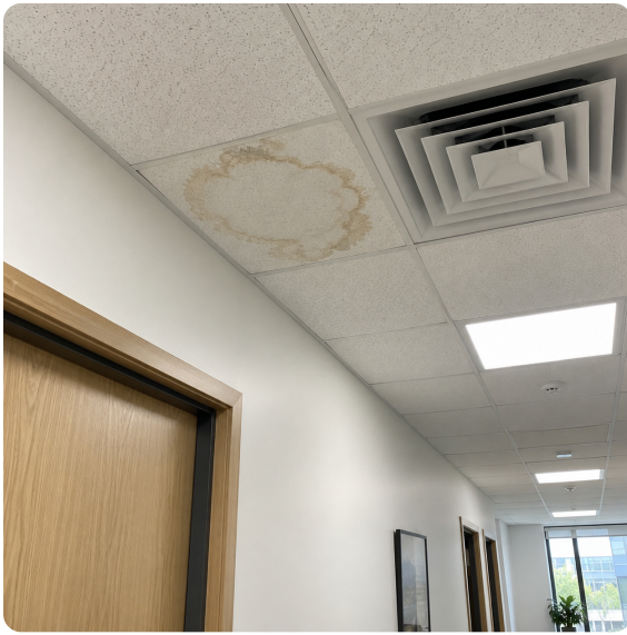
Level 2 - corridor outside Meeting Room 204
